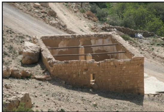
FIGURE 21: New roofing material, rail bars, used in the construct the prayer house at Shammakh
