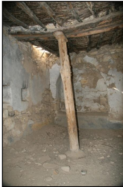
FIGURE 13: Wooden Posts supporting the roofs at Shammakh
