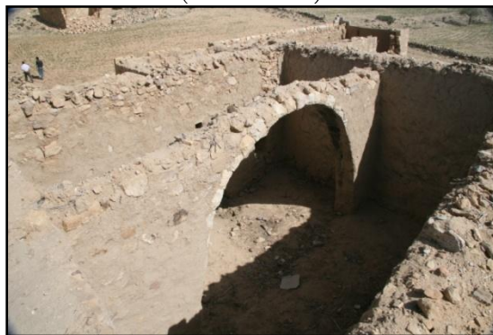
FIGURE 12: Roofing System based on Arches at Shammakh
