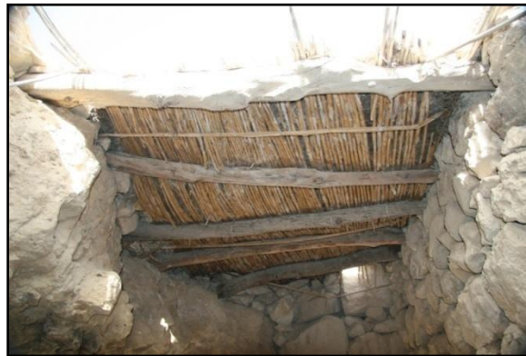
FIGURE 14: Wooden beams and reeds as Roofing materials Shammakh
