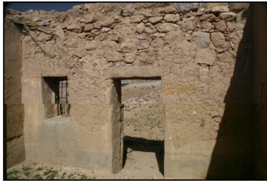
FIGURE 11: Details of coating technique and material
