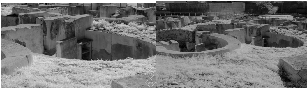
Fig. 4: Infrared photographs which differentiates between the original stone (in gray) from the reconstructed concrete (in white, this difference between these two materials is exaggerated through the reflection of sunlight).
